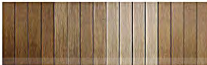
After Installation 2 Years After Use After Cleaning After Maintenance
